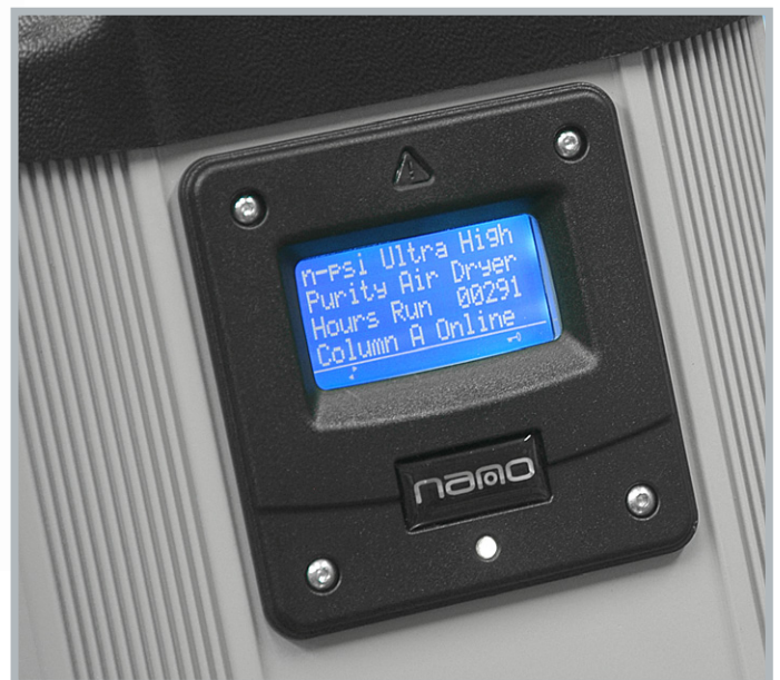
PLC controller with clear text display.
