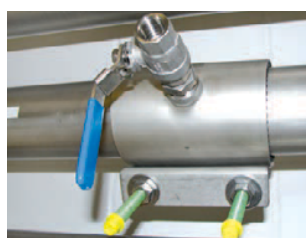
B Spot drilling collars
